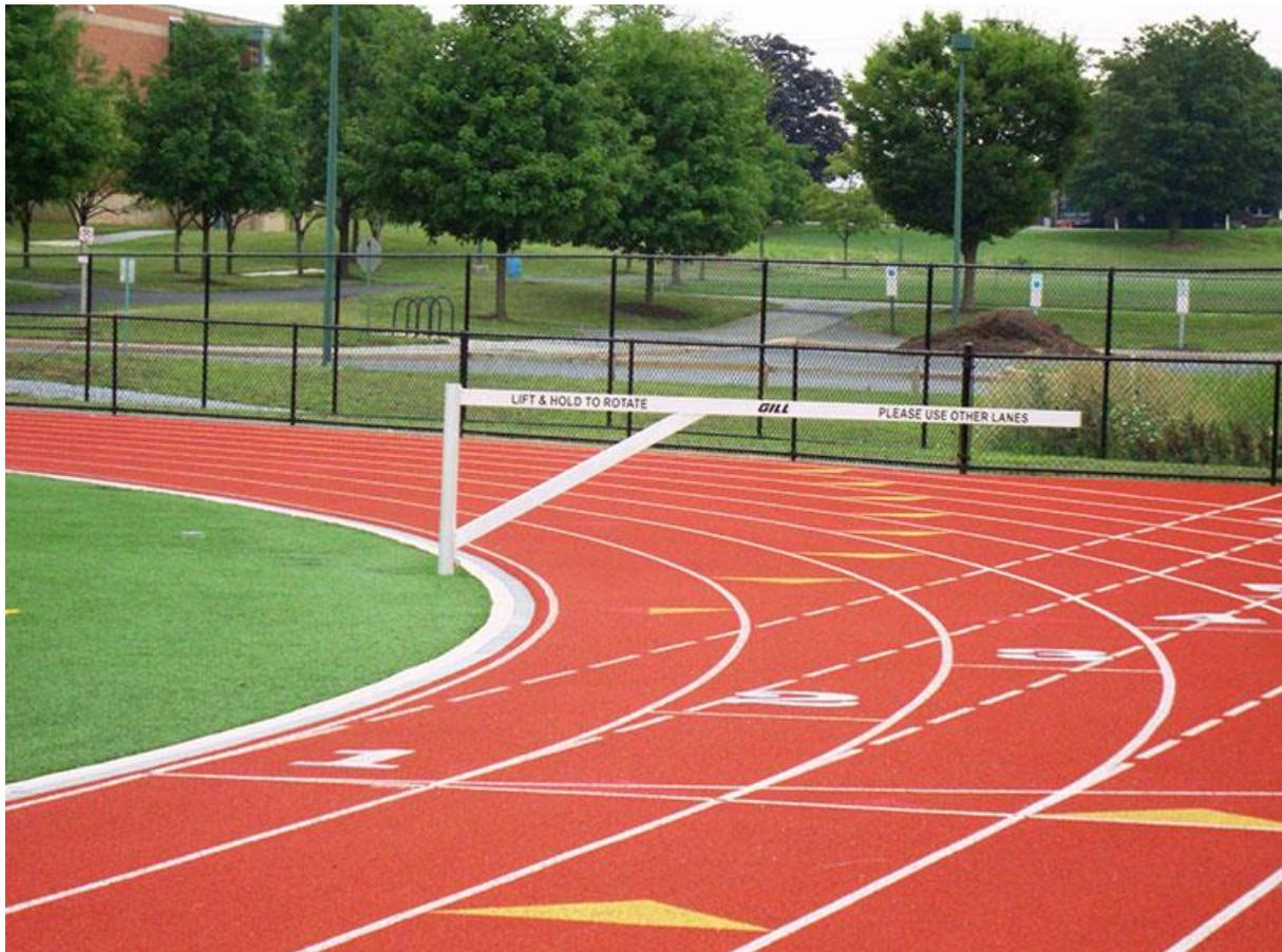
Experience shows that the inside two lanes of an athletics track suffer the disproportionate levels of wear and tear and, in order to protect the long term life of the track surface and prevent early (costly) remedial work, facility operators should explain this to track users / clubs and actively encourage the use of outer lanes during training/casual sessions.
